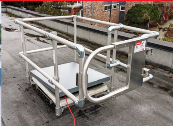
Guardrail for Roof Access Hatch
