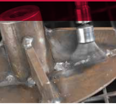
Cleaning hard-to-reach fillet welds on a gusseted base plate.
