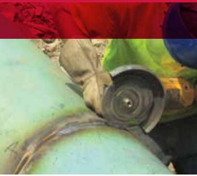
Removing weld slag before the next weld pass.
